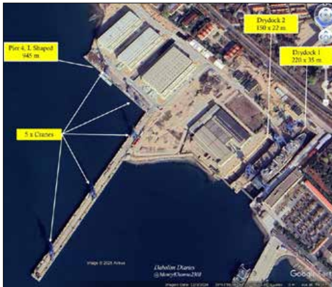
Figure 8: Ship Repair Facility as in 2024 (Google Earth 03 Dec 2024)
