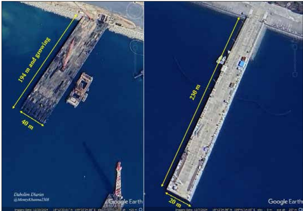
Figure 6: Dimensions of Piers at Probable 3rd Base (Left) and 2nd Base, Longpo (Right)
