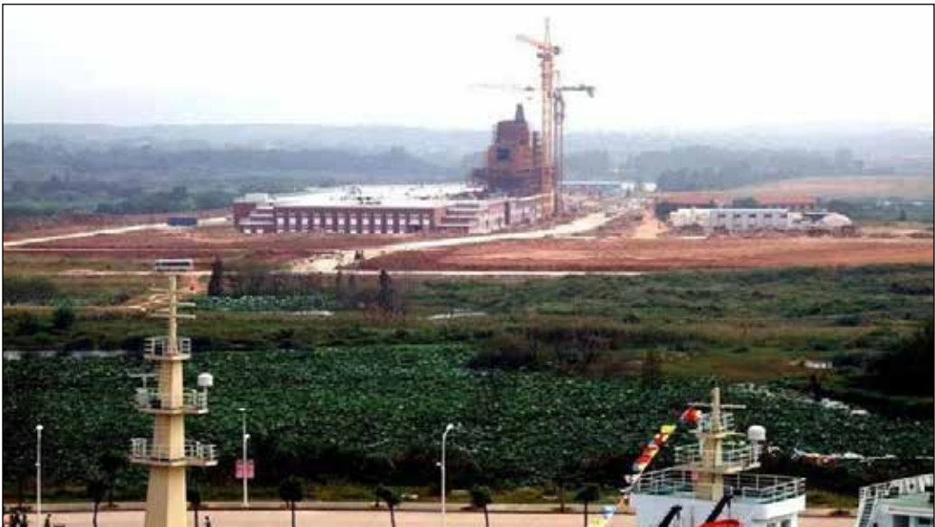
Figure 1: Full-Scale Mock-Up of Liaoning Under Construction at Wuhan
