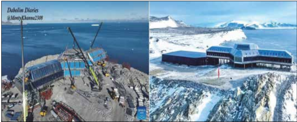
Figure 11: Qinling Station Under Construction (Left) and Completed (Right)
