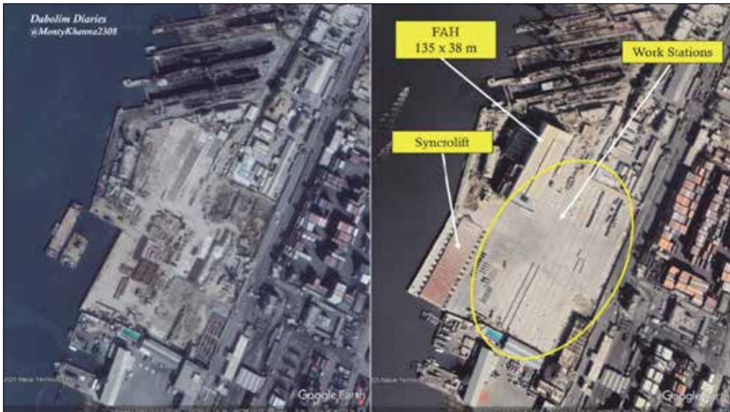
Figure 2: Ship-Lift and Transfer System at KS&EW. Google Earth Images dated 02 Nov 2018 (Left) and 08 Feb 2021 (Right)
