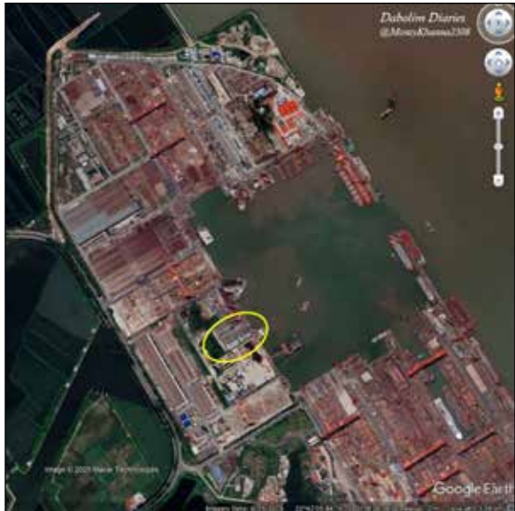
Figure 3: Zubr Class Facility on the Western Side of GSI (Circled)
