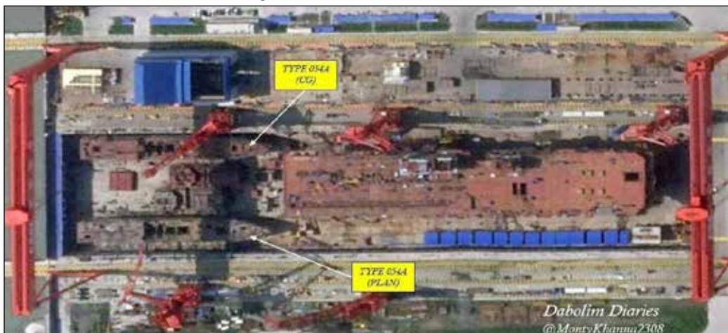
Figure 3: New HDZH Drydock
