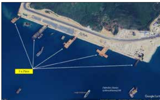
Figure 1: Construction Activity at Yulin Probably for a New Nuclear Submarine Base
