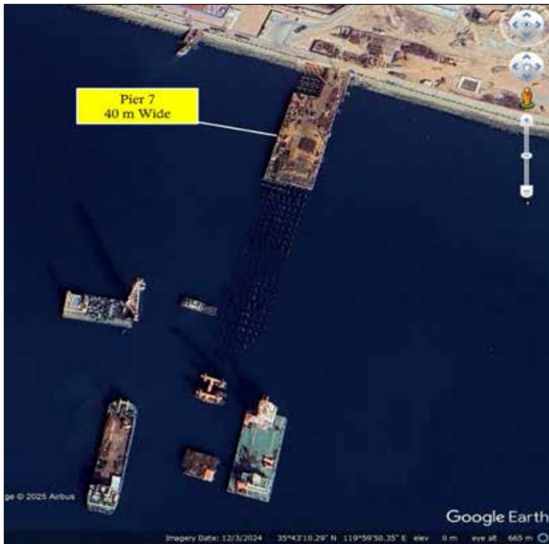
Figure 10: New Jetty (Pier No 7) under construction (Google Earth 03 Dec 2024)
