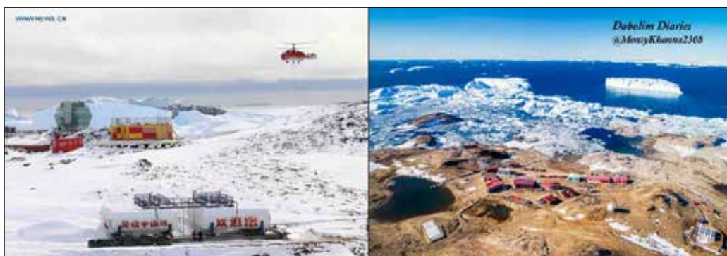
Figure 7: View of Zhongshan Station - 09 Feb 2019 (Left) and Contemporary Aerial View (Right)
