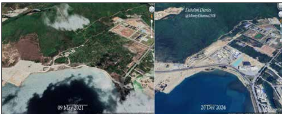
Figure 3: Creation of Administrative Infrastructure Adjacent to Piers
