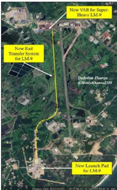
Figure 8: Launch Infrastructure for Long March-9 Under Construction at WSLC
