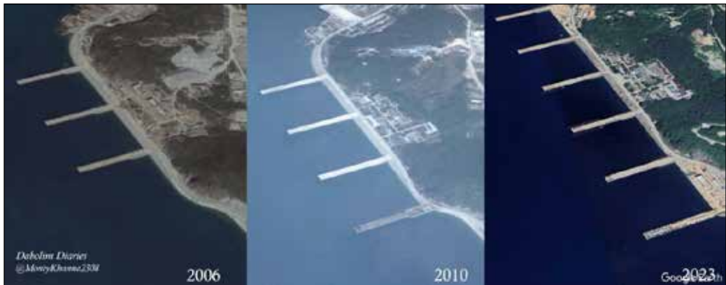
Figure 7: Phased Augmentation of Piers at 2nd Base, Longpo
