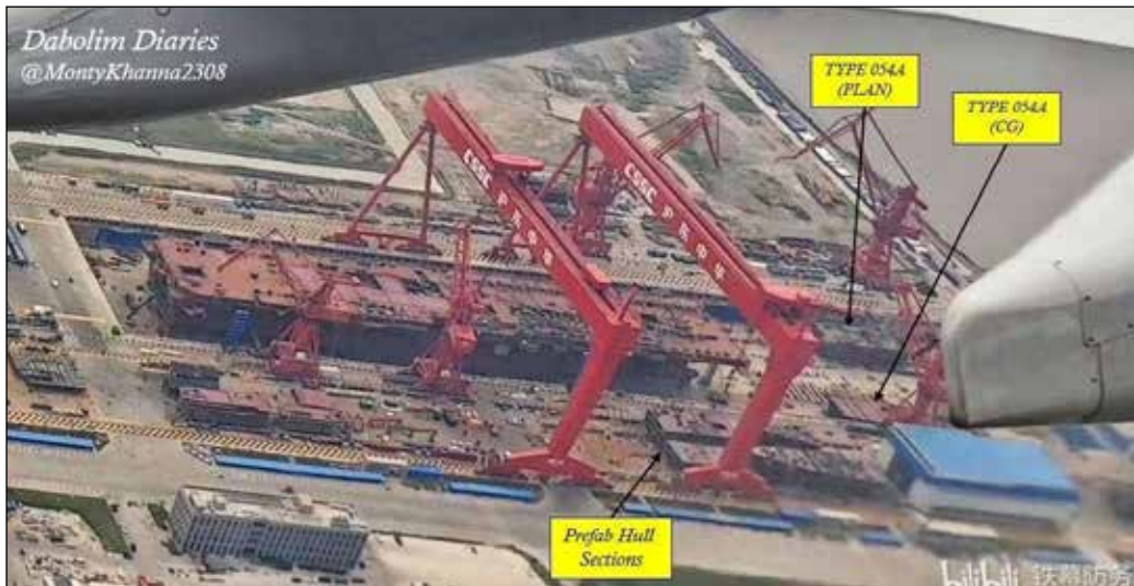
Figure 2: New HDZH Drydock
