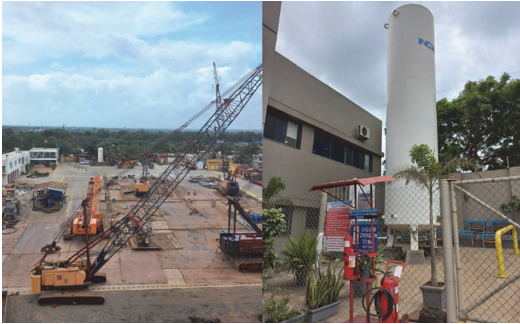
Figure 8. Geo-membrane layer on the yard and Liquid Oxygen supply tank in a yard
